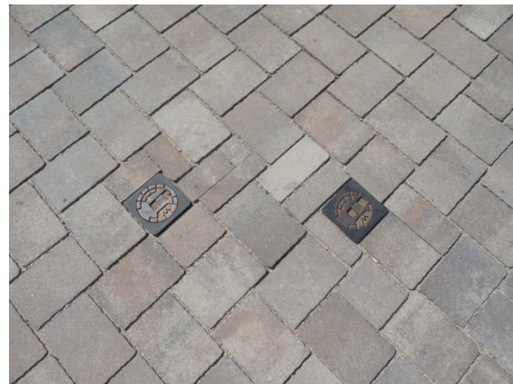
Surface box for pavement installed in pavement
