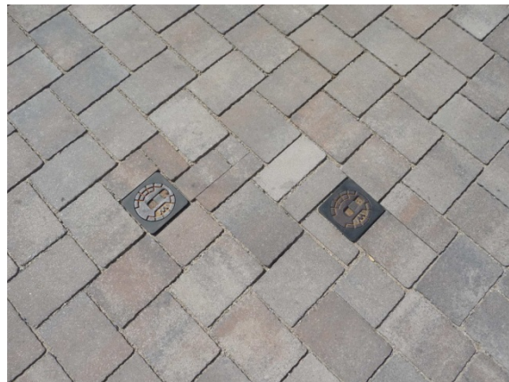
Surface box for pavement installed in pavement
